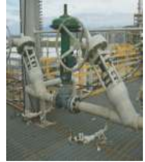
Globe Valve, Y type, Non Return, Pressure Seal RIO POL - LUMMUS SNAM PROGETTI
