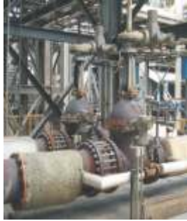
Gate Valve Bolted Bonnet and Dual Plate Check Valve 20" - 300# GRUPO COSAN - DEDINI
