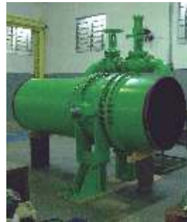
Butterfly Valve 40" with by-pass for Small Hydroelectric plant ENERG POWER
