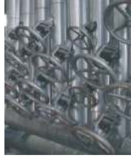
Severe Service Stop-Globe Valve (Durblock) ARACRUZ
