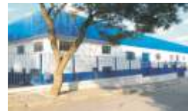
Serial-made Valves Cajamar - SP - Brazil
